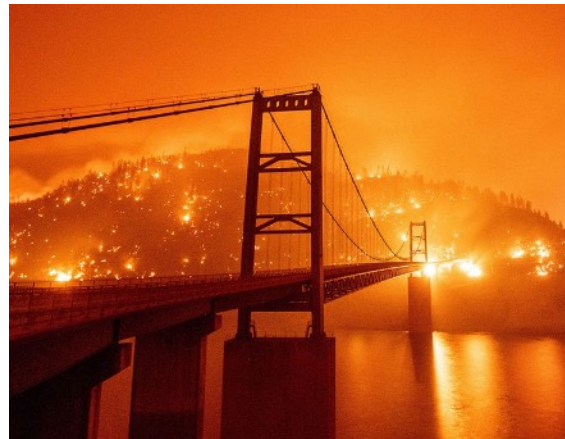
Wildfire in the vicinity of the bridge
