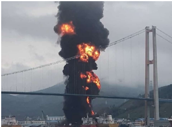
Industrial fire below the bridge deck
