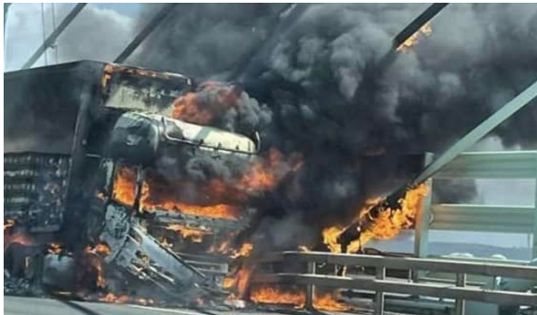
HGV fire on bridge deck
