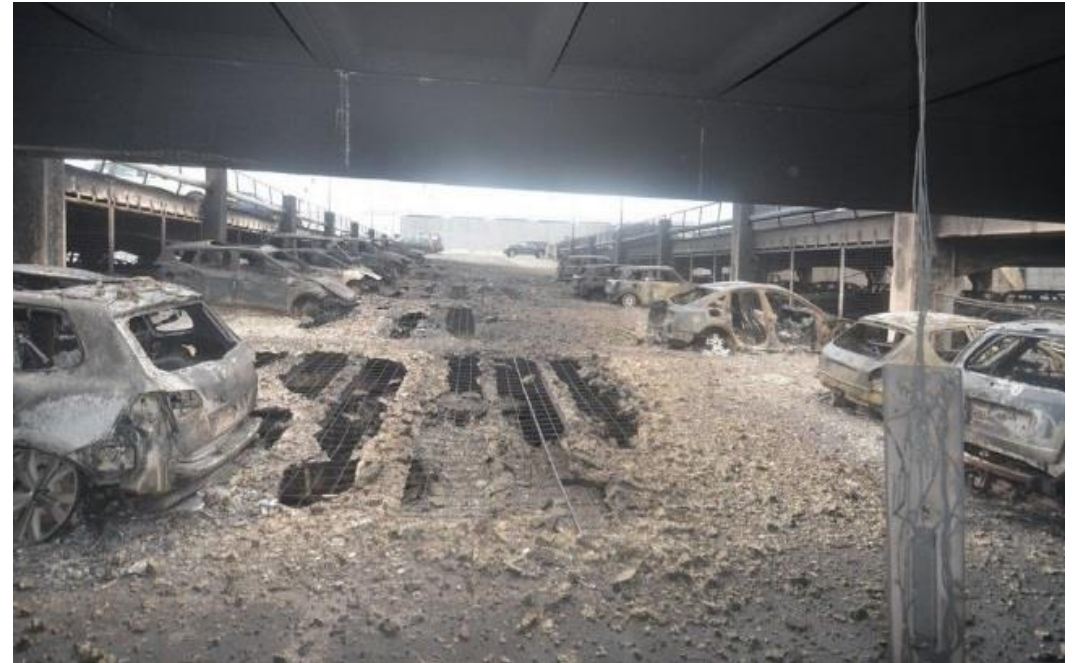
Disintegration of floor slab. Image courtesy of MFRS.
