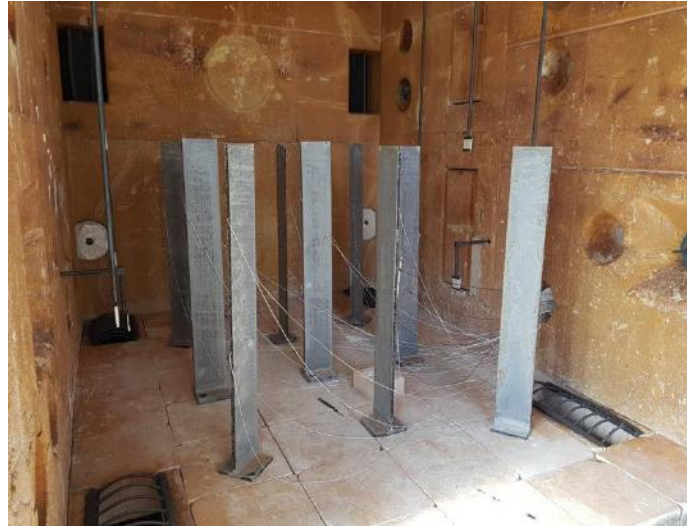
Test specimens after the fire test
